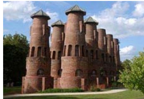
Denise Sanchez/Morning Call via AP Old cement kilns are located in Saylor Park in Coplay, Pa. The century-old kilns owned by the first American producer of Portland cement might be torn down because the county that owns them says it can no longer afford their upkeep.
